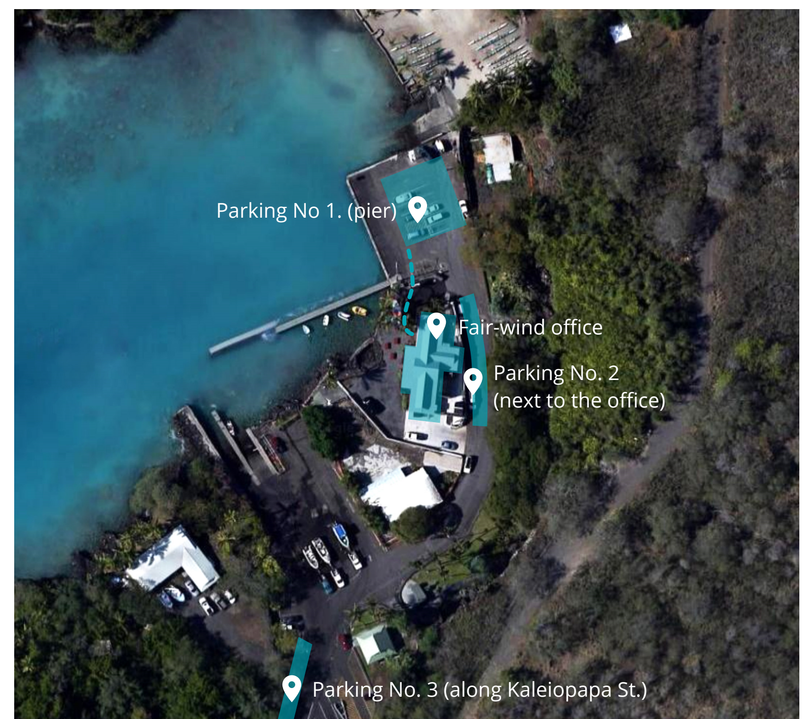
Parking No. 1. (pier)
